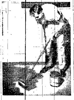
Rolling paint on floors with a long-handled paint roller saves time and effort. It's good tool for painting ceilings, too.
